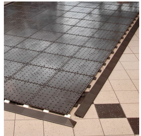
Finish platform with tapered frames / edging
